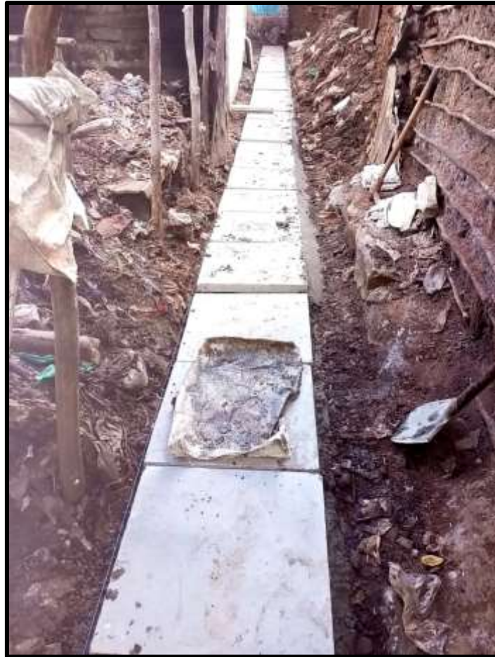
Sewer lines are improved and covered all around the centre (August 2021)
