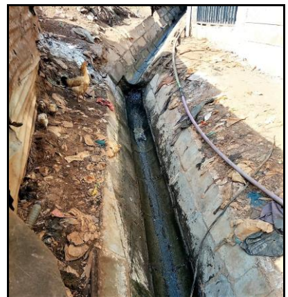
Improved sewer lines
